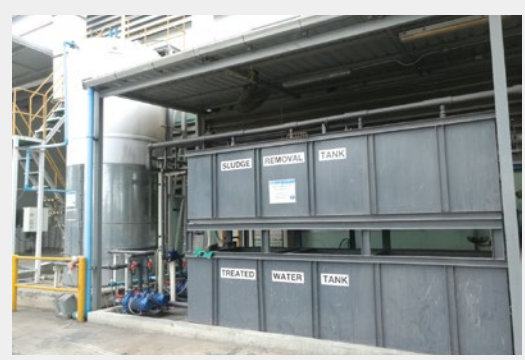
Painting wastewater treatment equipment
