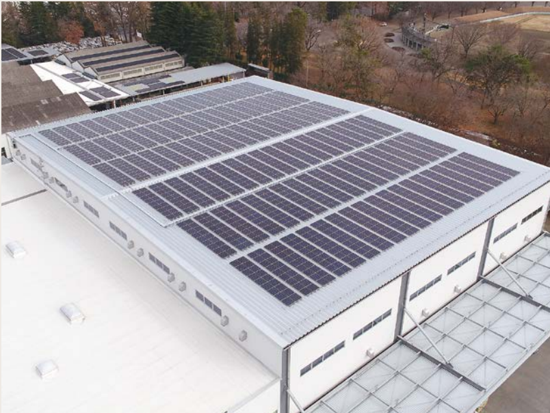
Solar panels installed on the factory roof
