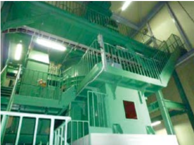
This giant crusher has 2.4 times the processing capacity of the previous equipment
