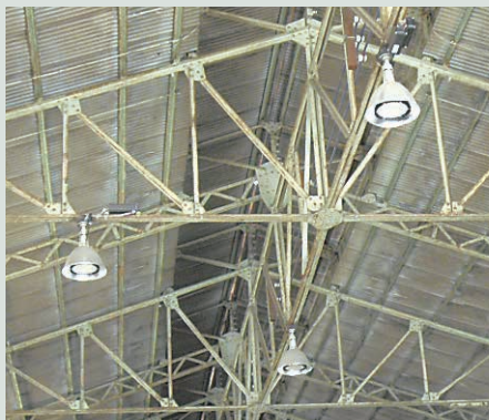
High-ceiling LED fixtures
